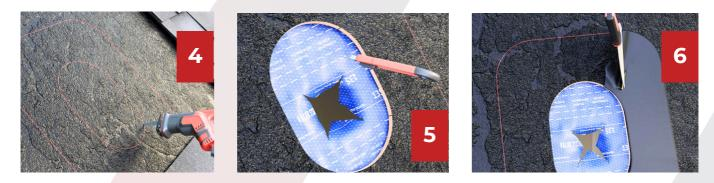
4. Clean the surface around the opening and then apply sealing (roofing sealant - not included) to the prepared surface (pic. 6). Evenly press the base and then fasten with roofing nails through the predrilled holes (pic. 7).
